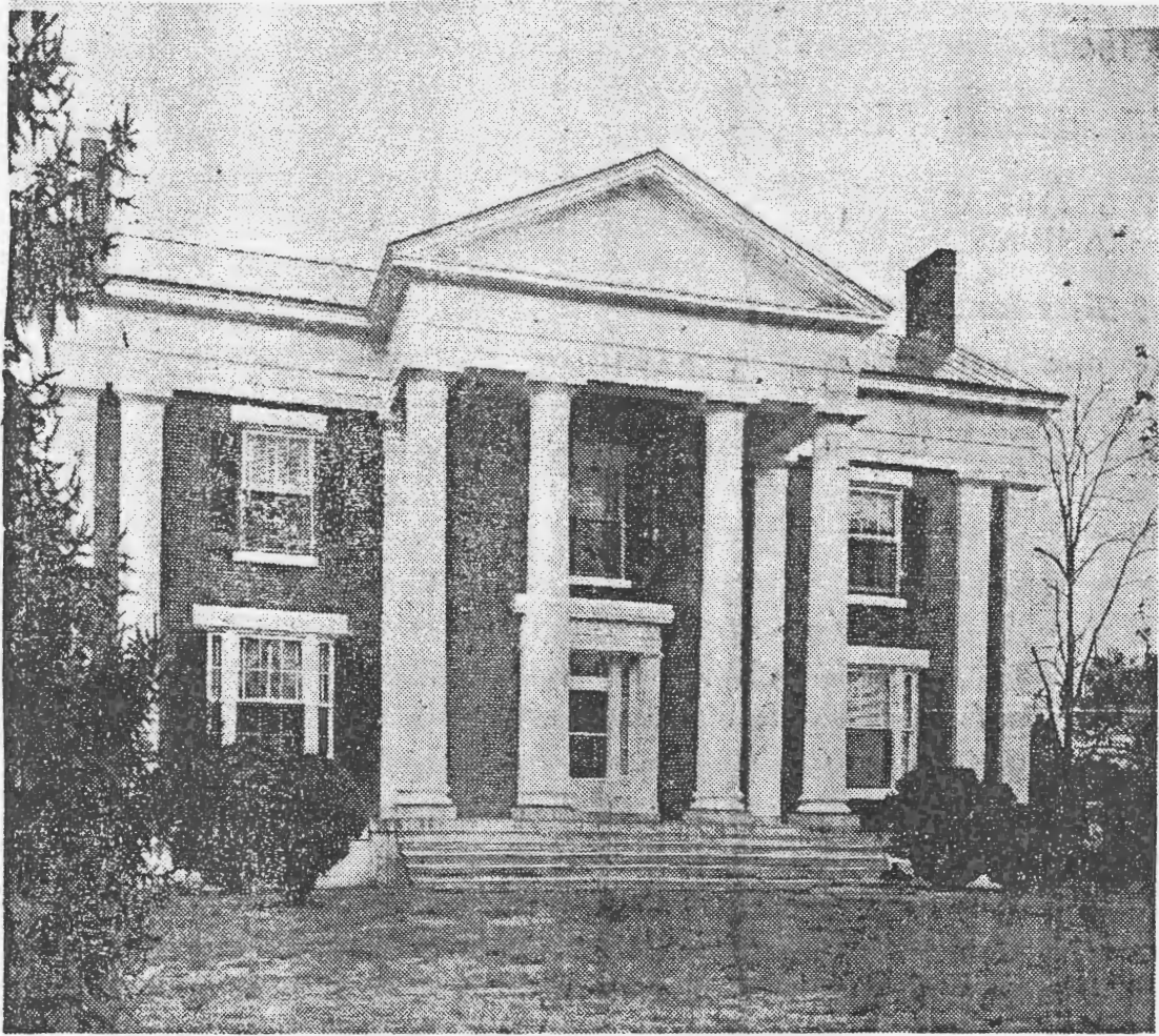
ROMAN DORIC —Built in the 1840's, the house is a Roman Doric example of Greek Revival architecture. It has ash floors, double poplar and single walnut doors downstairs, poplar woodwork upstairs.
